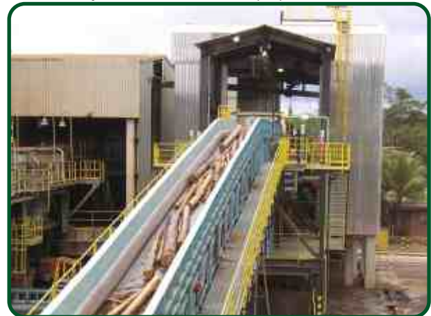
Cenibra Project, Belo Oriente / MG pulp mill.
