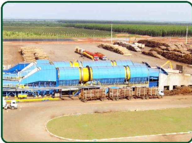
**D**EMUTH woodhandling comprises two chipping lines with drum debarkers, chip screening station (2 chip selecting screens with 1.000 m<sup>3</sup>/h capacity each), bark chipping station, storing and many conveyors (more than 2.500m long).
