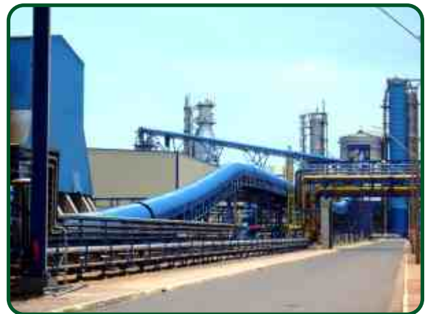
Horizonte Project, Fibria mill in Três Lagoas/MS.
