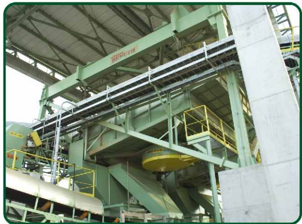
Bahia Pulp Project, Bahia Pulp Mill in Camaçari / Ba.
