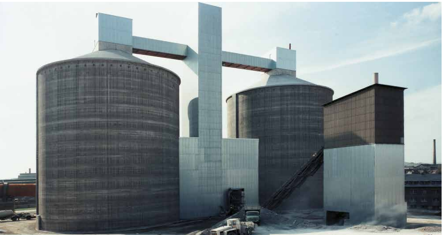
Clinker Silos 2 x 60,000 t
