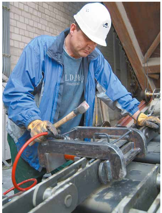
Pre-assembly of chain strands
