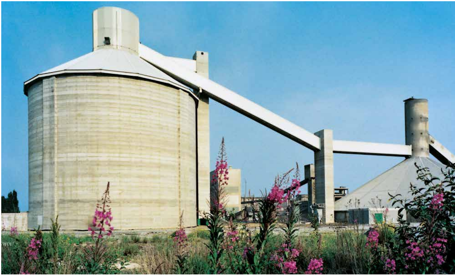
80,000 t silo with steel roof
