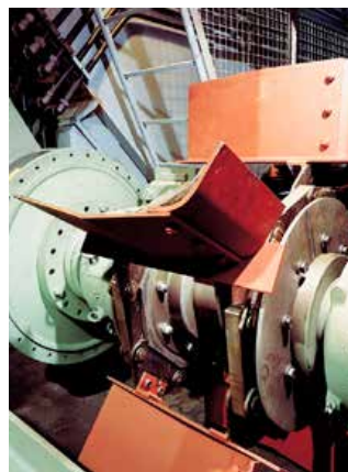
Scraper chain drive
