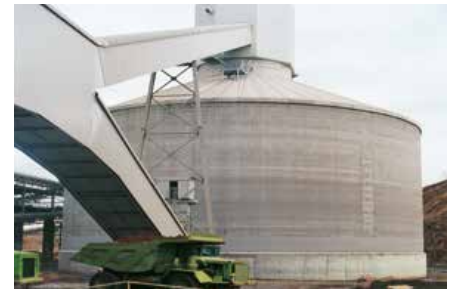
Circular storage hall with internal silo and earth cone
