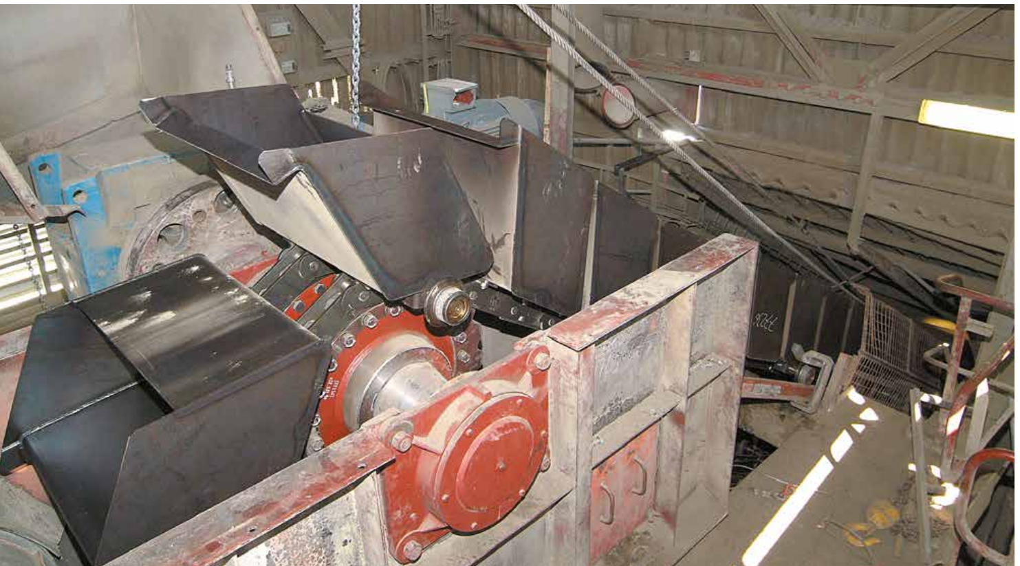
Installation of new bucket strand
