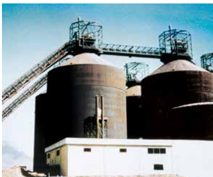
Steel silos, 30,000 t each
