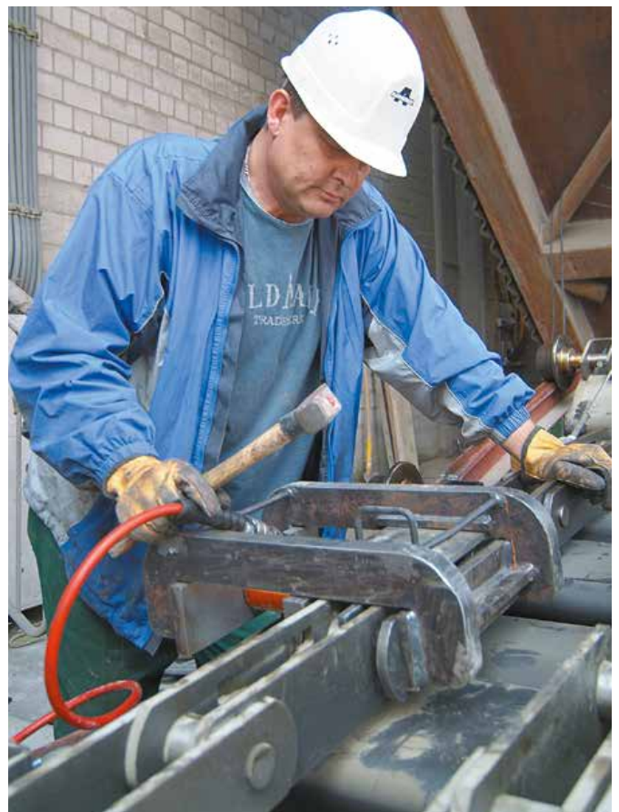
Pre-assembly of chain strands
