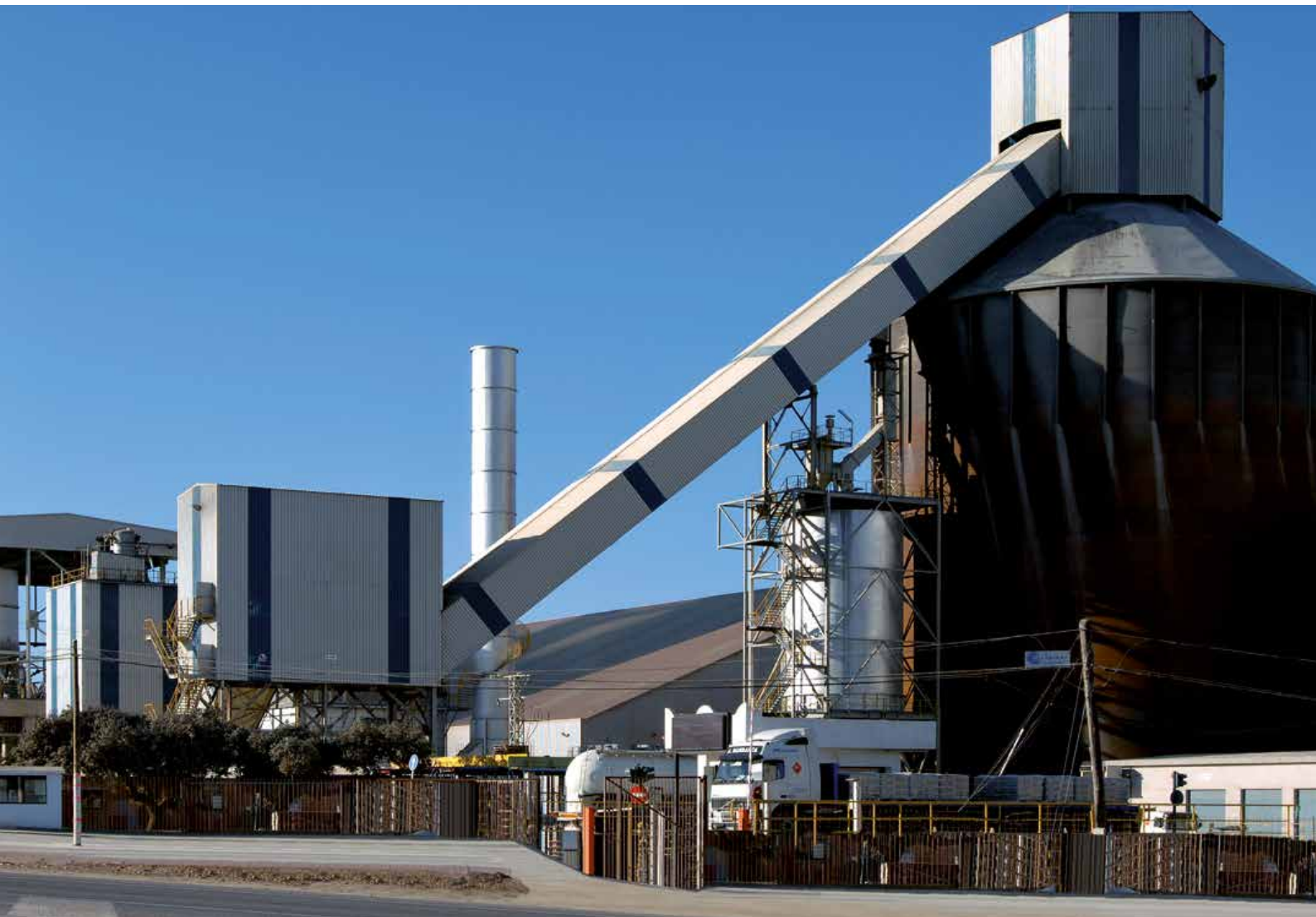
Pan Conveyor KZB-Q connecting cooler and silo
