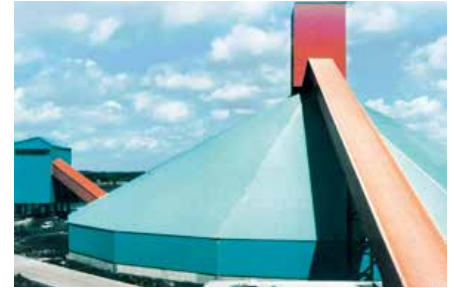
Covered stockpile with MOLEX®
