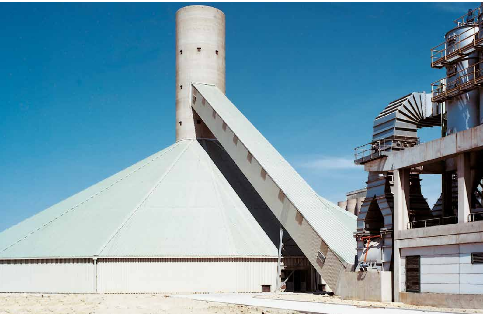
Feeding of covered stockpile
