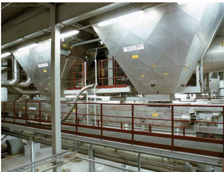
Hot boiler ash from a row of boilers
