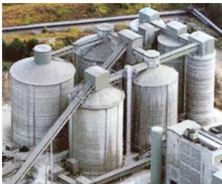
Silo group for different clinker types
