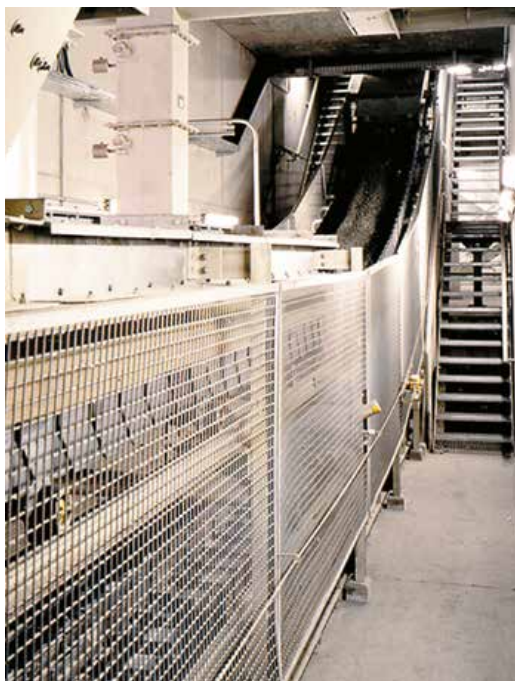
Deep Drawn Pan Conveyor under Clinker Cooler
