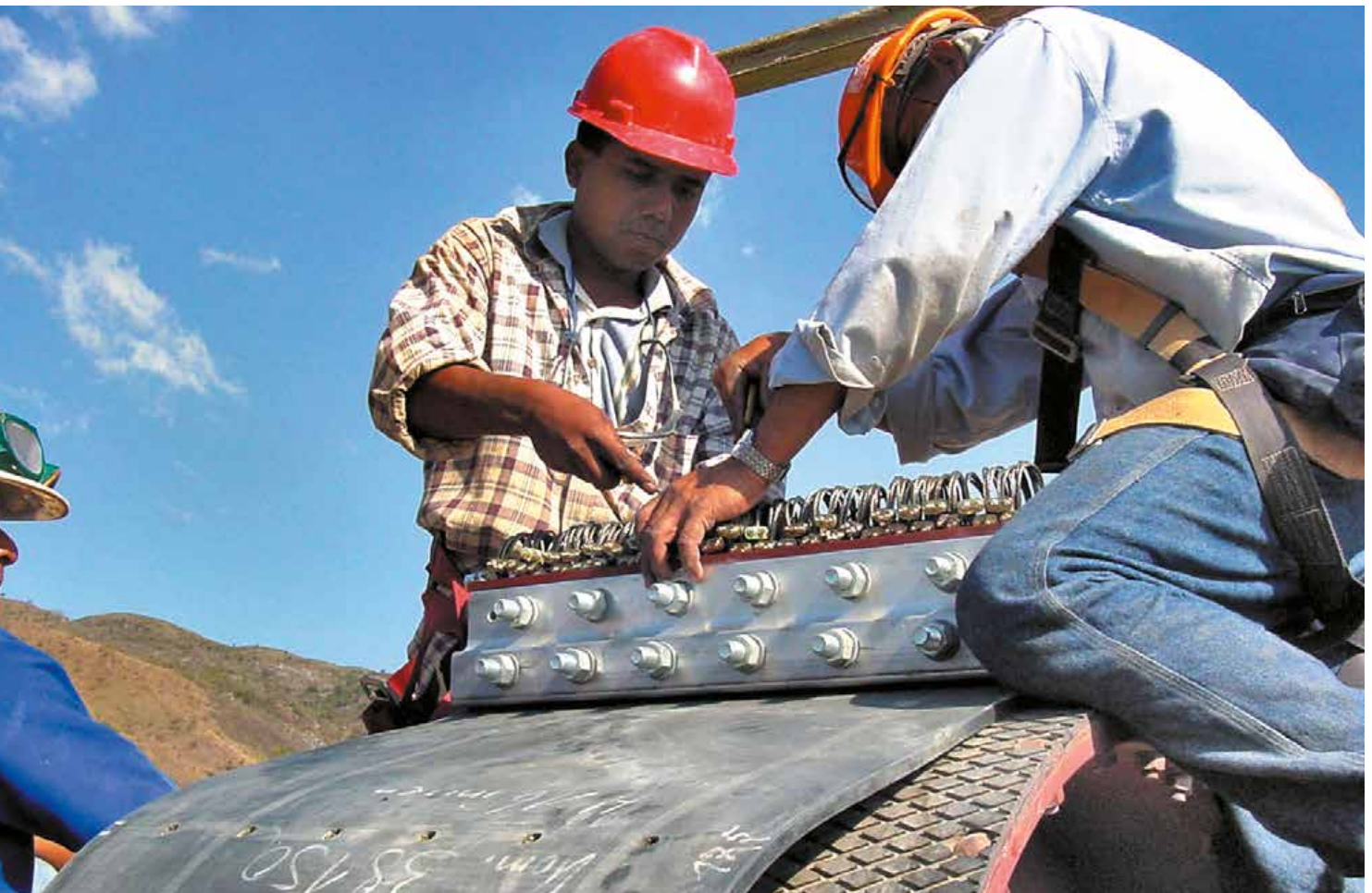
Splicing of steel-reinforced belt
