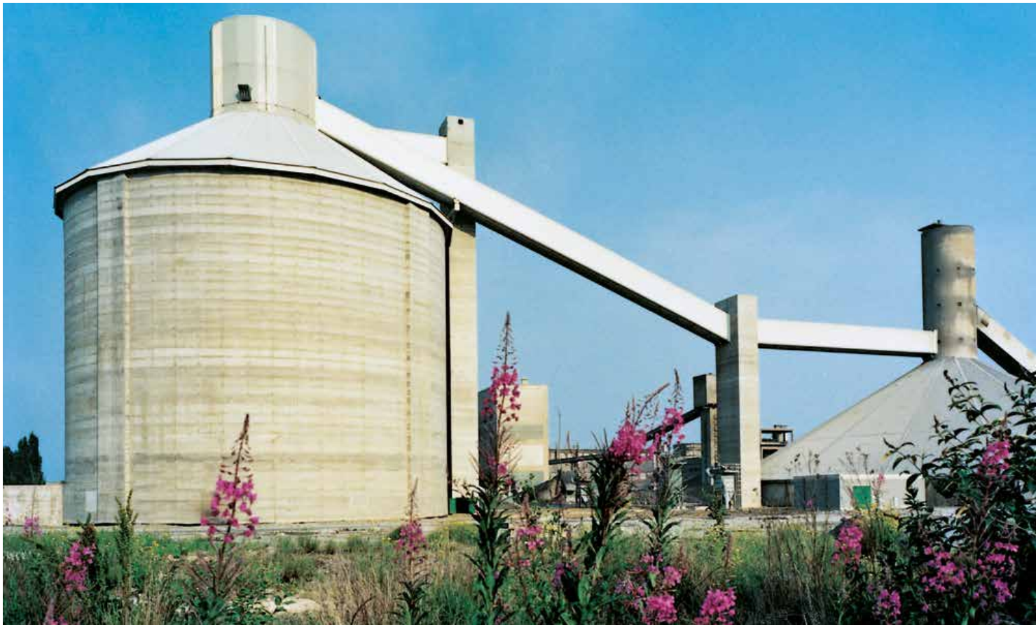
80,000 t silo with steel roof
