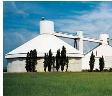
Circular storage hall 60,000 t
