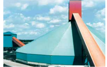
Covered stockpile with MOLEX®
