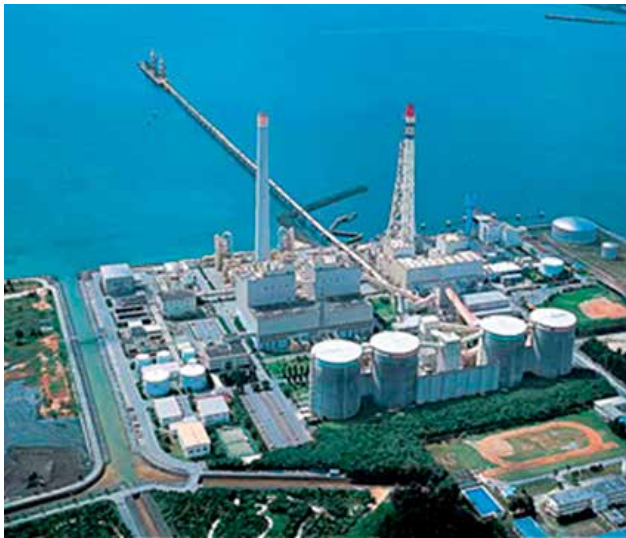
Denpatsu coal-fired power plant
