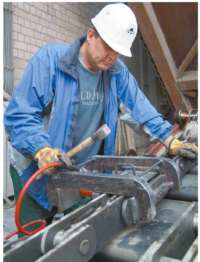
Pre-assembly of chain strands
