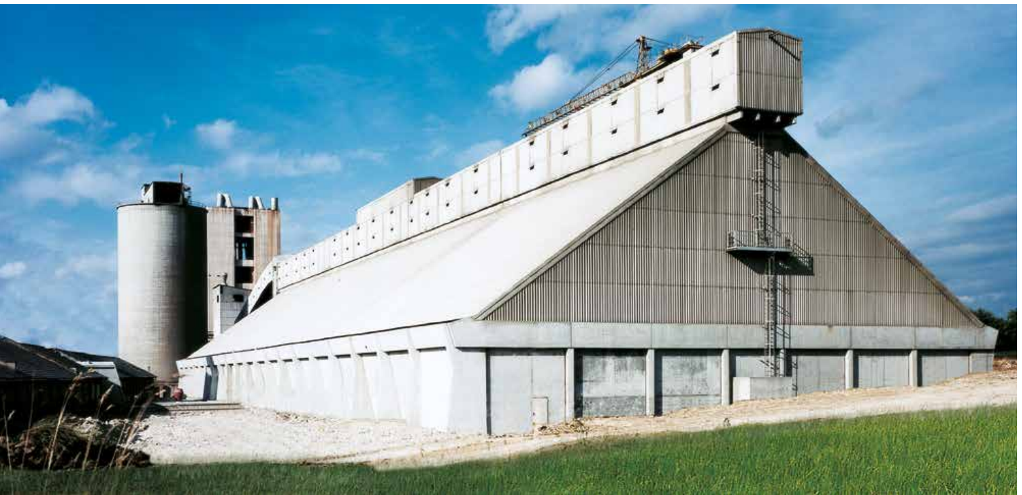
Clinker storage hall with earth cone
