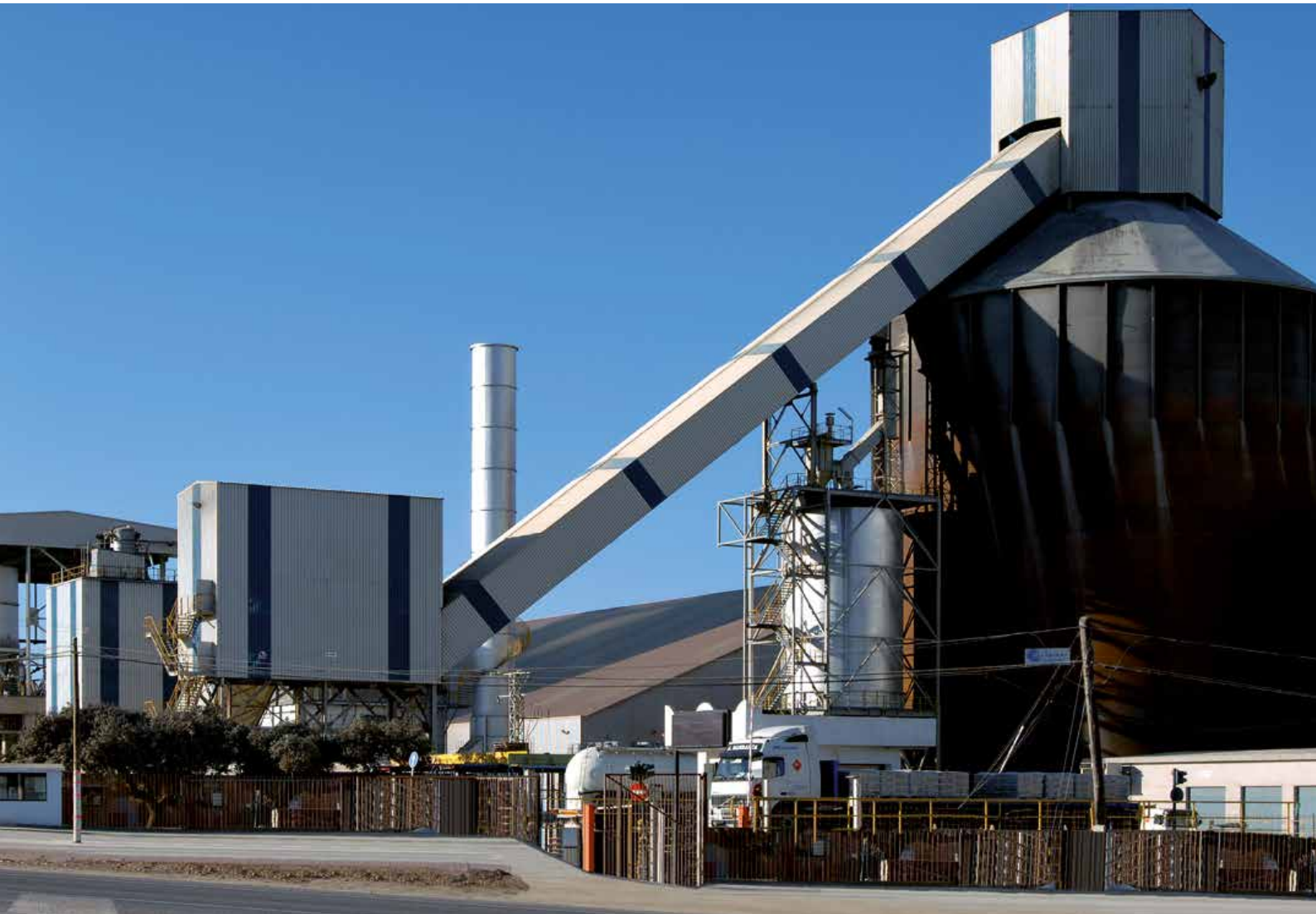
Pan Conveyor KZB-Q connecting cooler and silo
