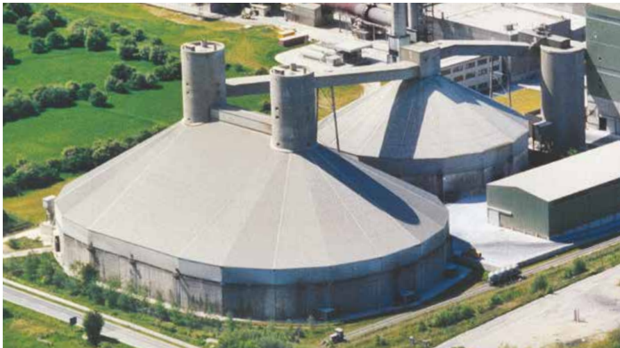
Oval storage hall with internal silos
