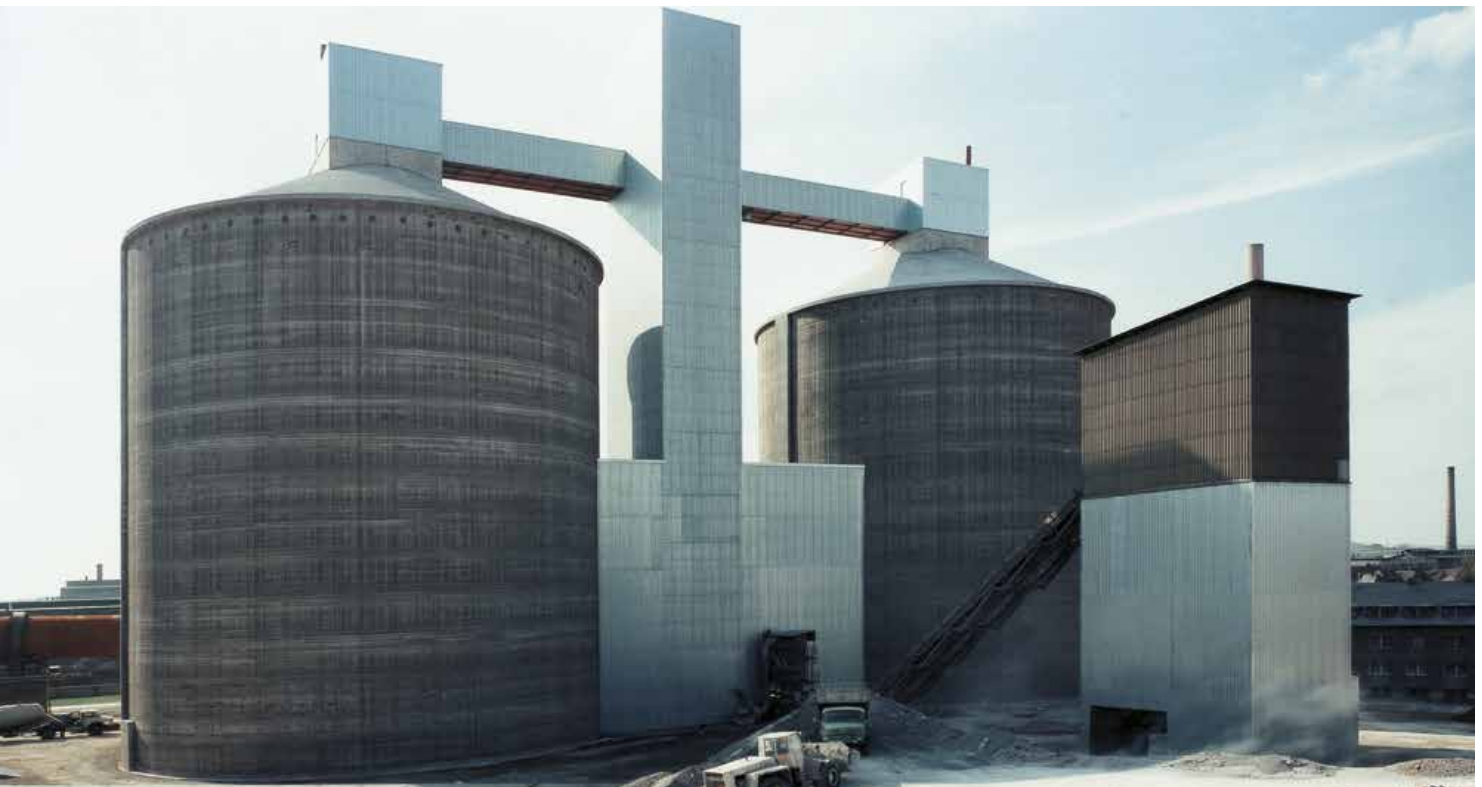
Clinker Silos 2 x 60,000 t
