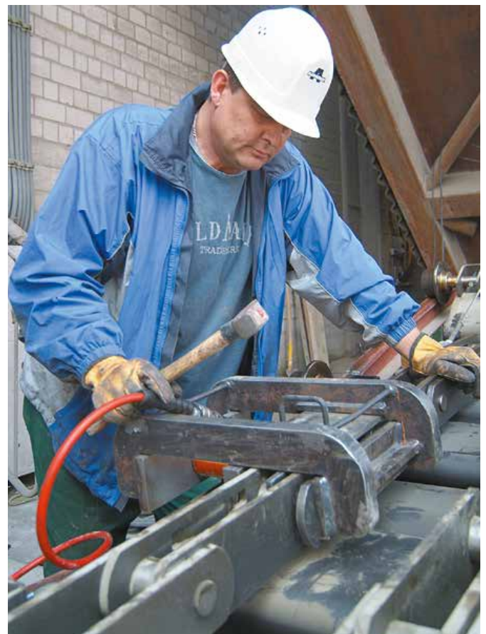
Pre-assembly of chain strands
