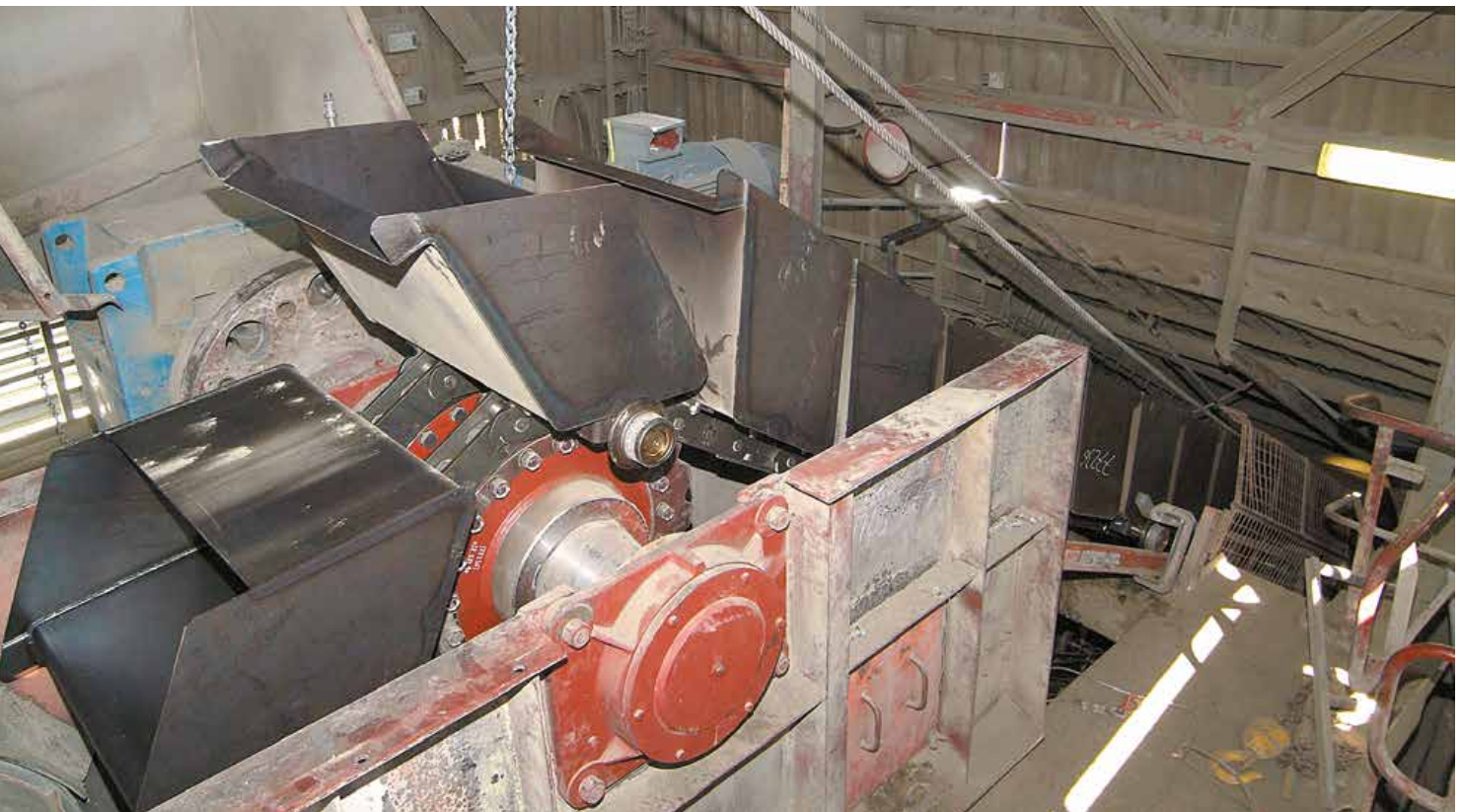
Installation of new bucket strand
