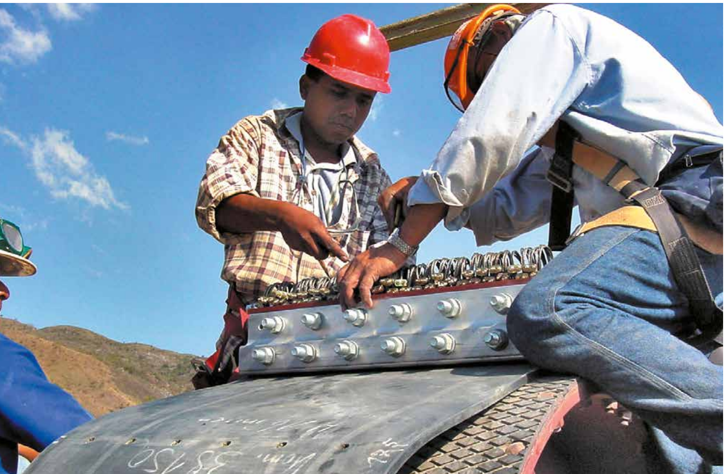
Splicing of steel-reinforced belt
