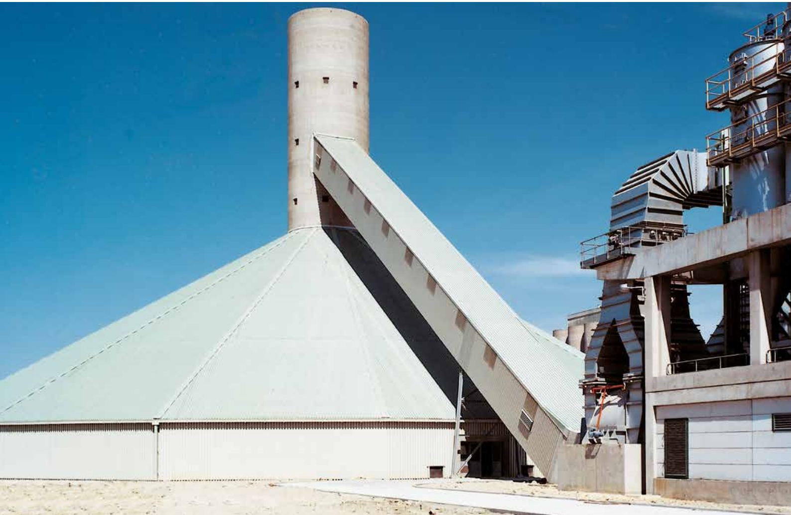
Feeding of covered stockpile
